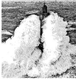
Because of its dangerous location and tumultuous engulfing waves, the beacon was started in 1904 but was not finished until 1911. Its foundation was hewn in solid rock and barely stands out of the water. There are times that the 154-foot-tall tower is lambasted by 65 to 97-foot waves. Many pictures have been taken of the lighthouse boldly standing with waves appearing to cover the beacon completely.
